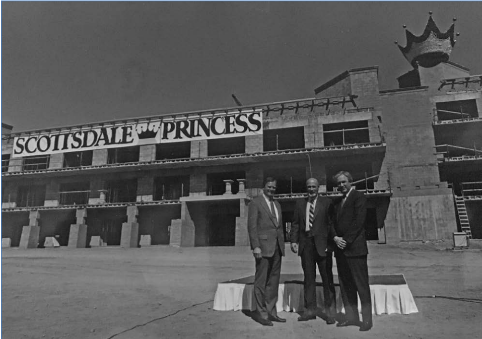
The Scottsdale Princess Resort celebrated its 'topping off' on March 3, 1987 as a crown was lowered onto its roof. Left to right: Manfred Gerling, Scottsdale Princess General Manager; Mayor Herb Drinkwater; John Price, President of Princess Hotels International, Inc. Scottsdale Area Chamber of Commerce collection
