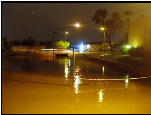
GRW north of McDowell Rd (Storm Date: 8/24/06)
