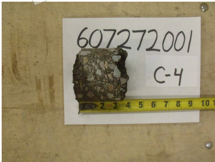
Photograph 10: Core Location C-4, asphaltic concrete thickness approximately 3.5 inches. Approximately 7.5 inches of aggregate base at C-4
