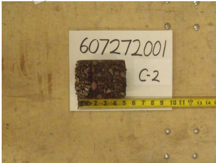
Photograph 8: Core Location C-2, asphaltic concrete thickness approximately 5 inches. Approximately 6.5 inches of aggregate base at C-2.
