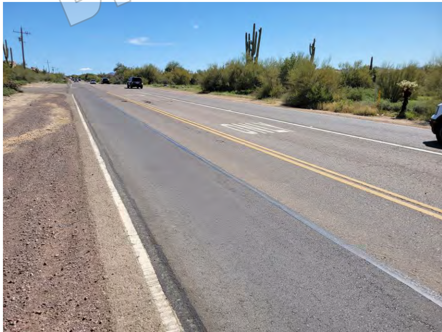
Photograph 6: Example of utility trench patch.
