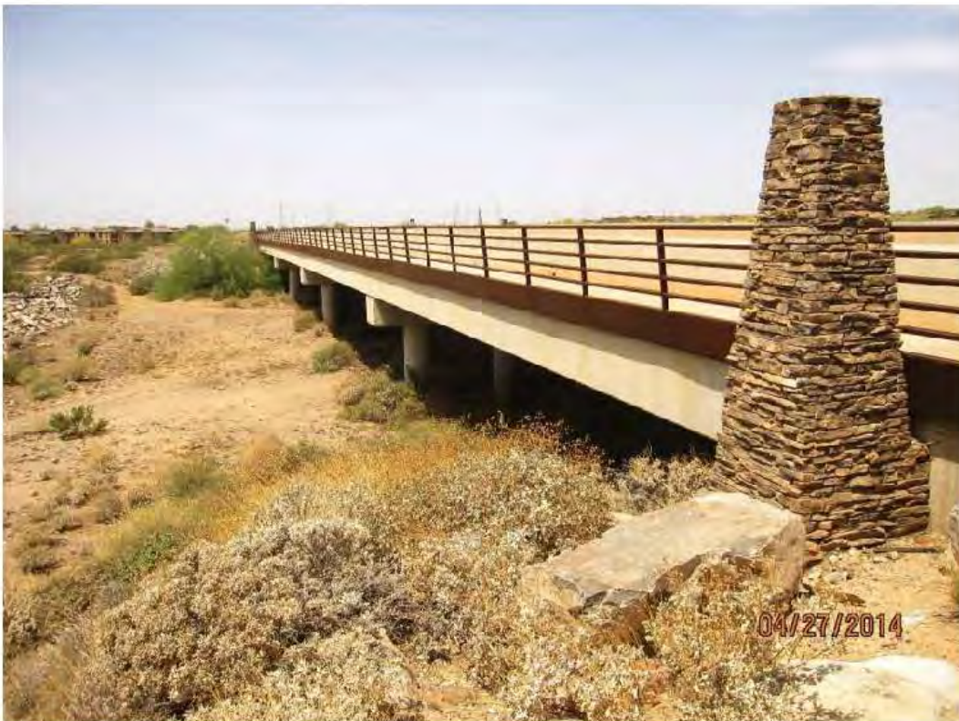
Upstream face of Bell Road Bridge
