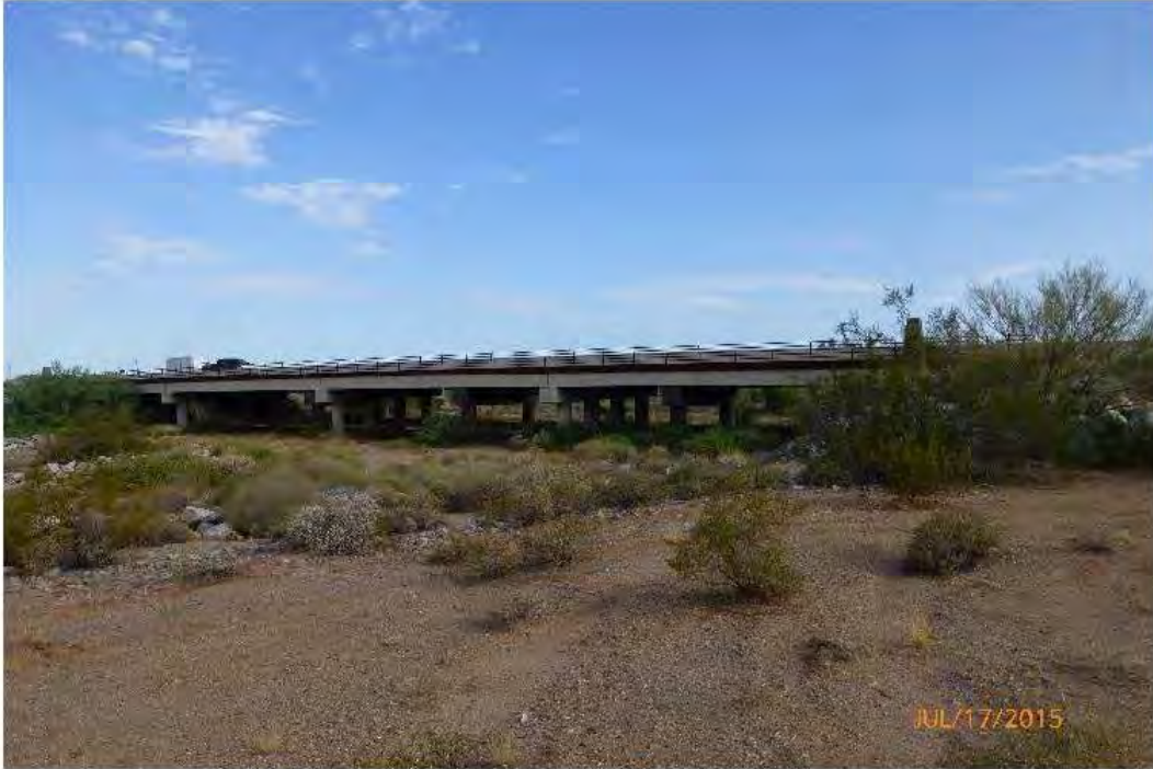
Downstream looking upstream at Bell Road Bridge
