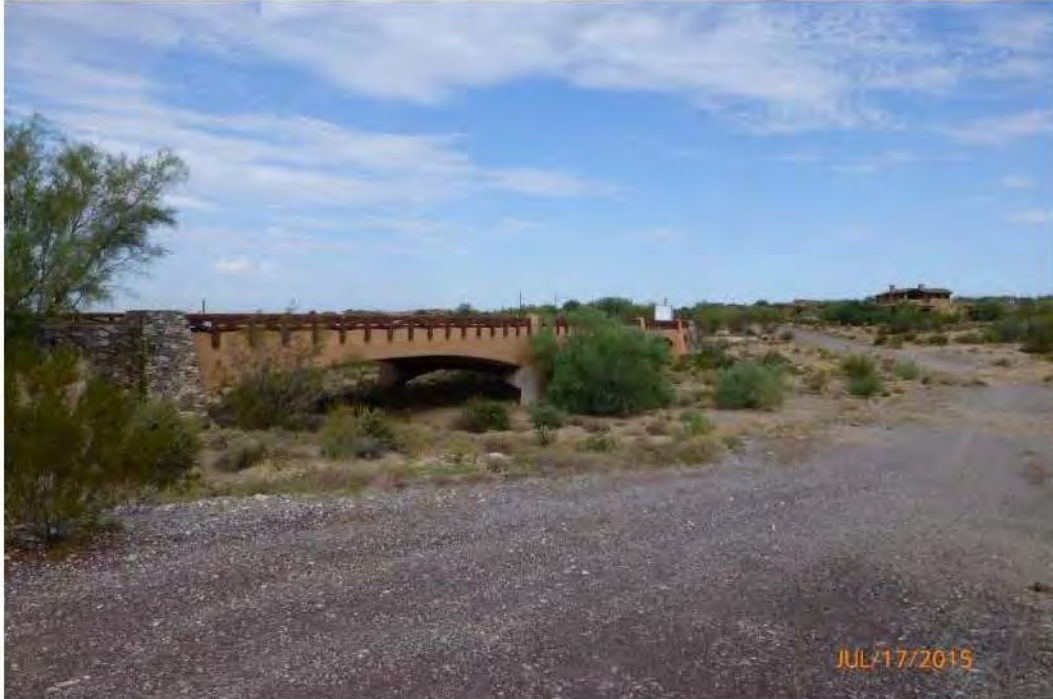
Looking at upstream face of Thompson Peak Parkway Bridge
