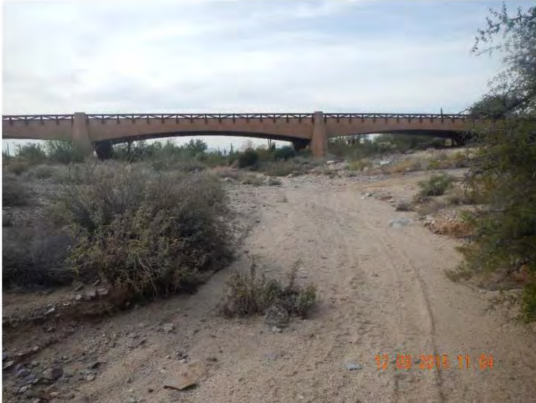
Downstream looking upstream at Thompson Peak Parkway Bridge
