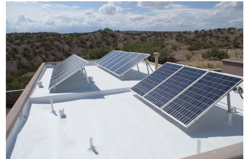
Credit: Carlisle Roof Foam
