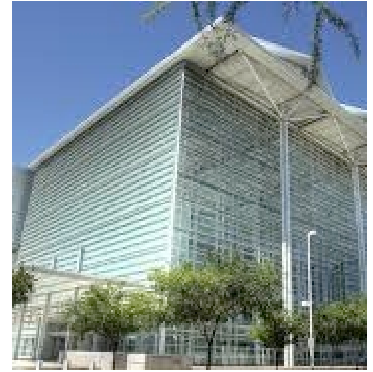
Federal Courthouse Phoenix - 2000 Glass & Steel - 25 years
