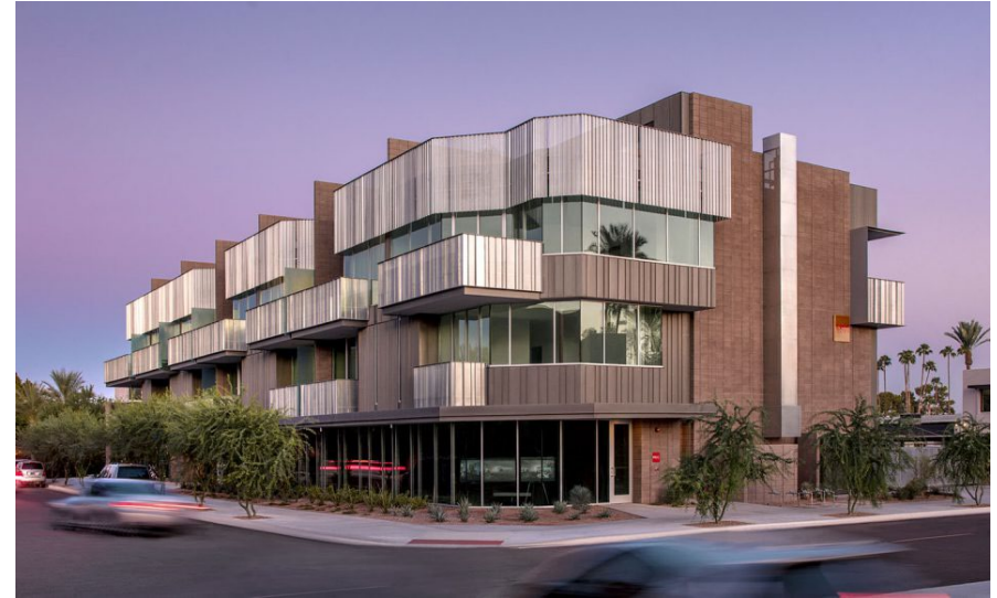
Eldorado on 1 st Condos – Will Bruder Architects
