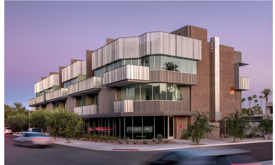
Eldorado on 1 st Condos – Will Bruder Architects
