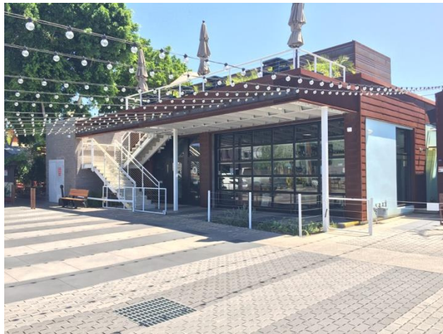
Creative Center – IgCC Compliant (2016)
