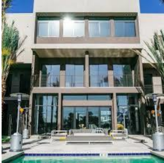
Equinox – IgCC Compliant (2016)
