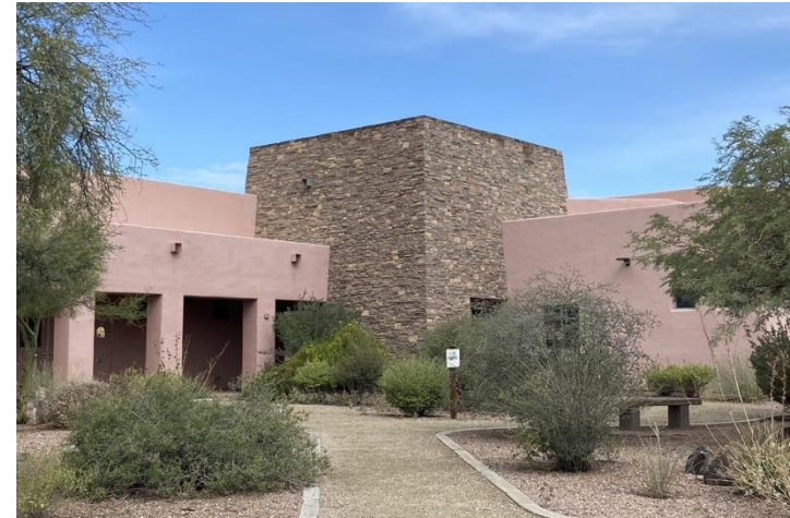
Papago Buttes Church of the Brethren Insulated Concrete Forms Walls (2005)
