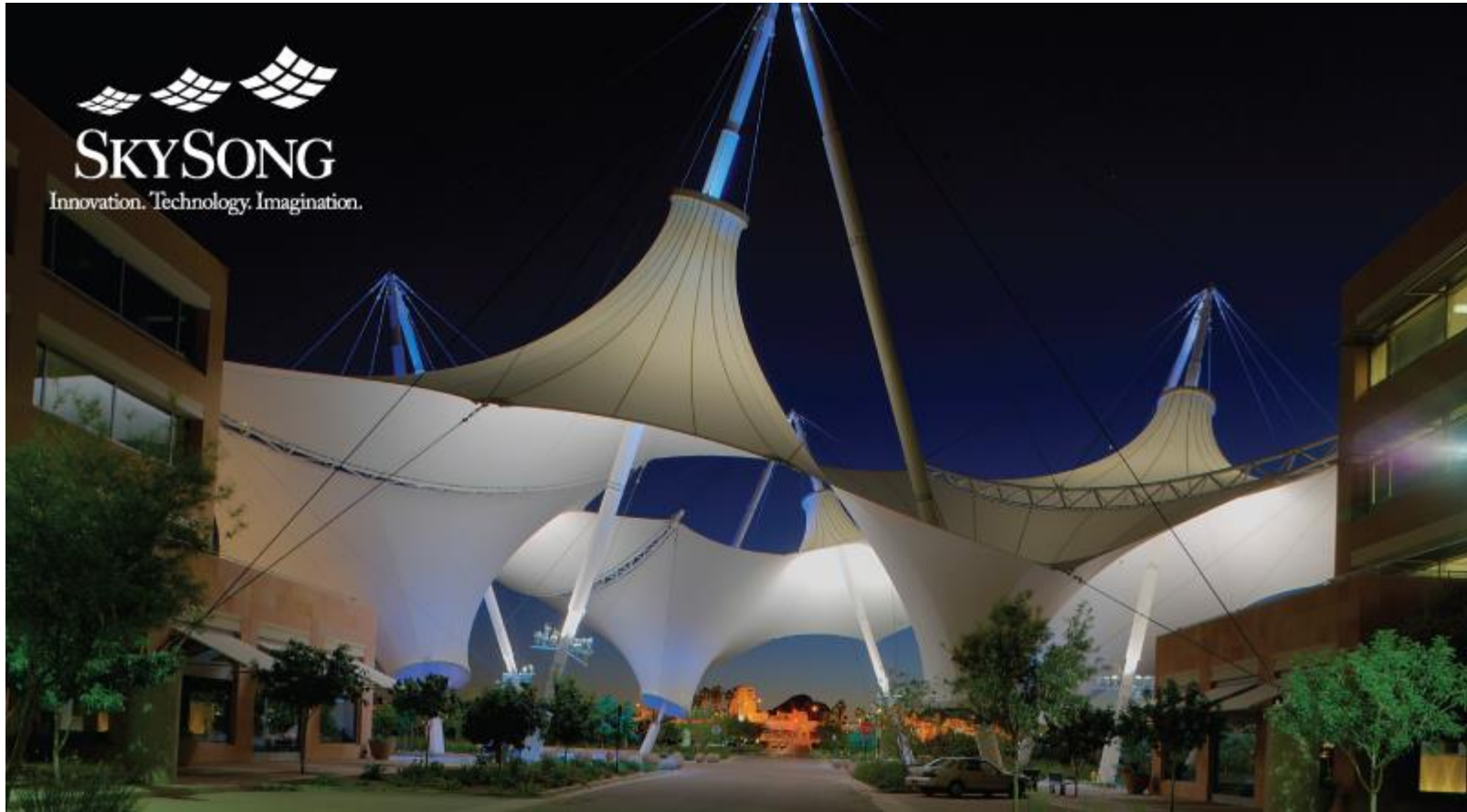
ASU Scottsdale SkySong Innovation Center Buildings 1 & 2 LEED Silver certification (2008 and 2009)
