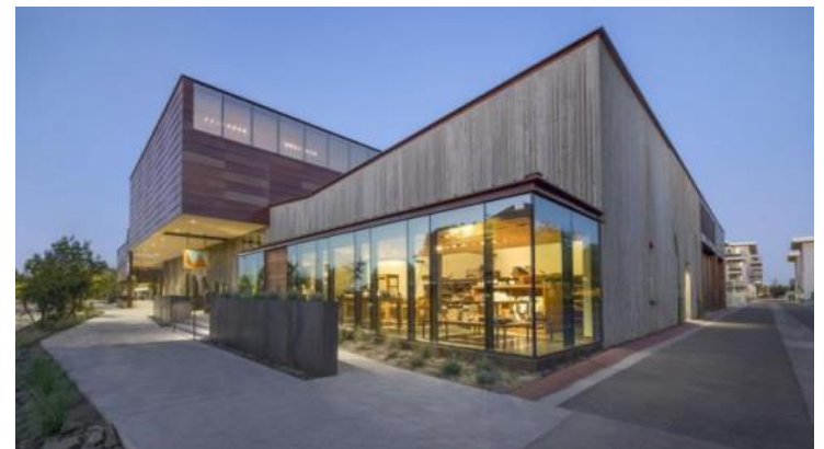
Museum of the West – LEED Gold
