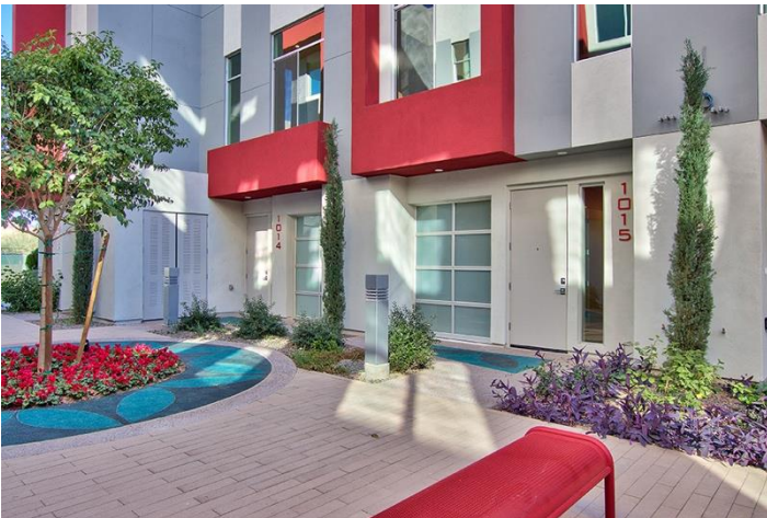
SOHO Townhomes – IgCC Compliant (2020)
