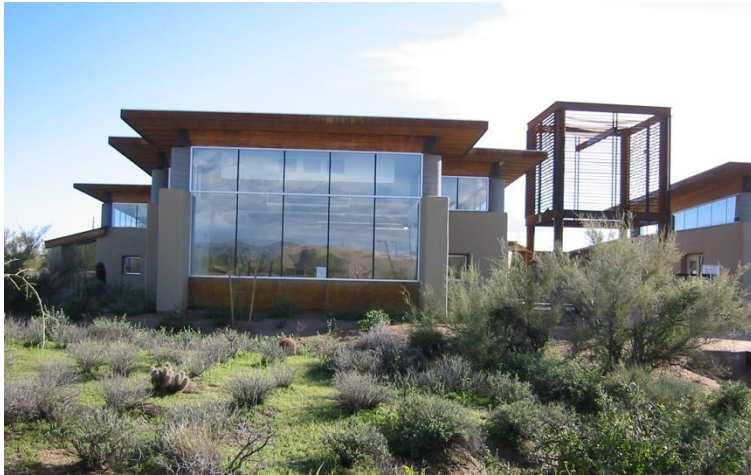
Foothills Academy – Weddle Gilmore Architects Strawbale constructed walls (2002)
