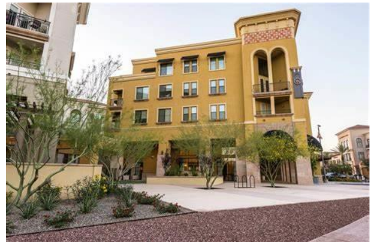
Broadstone Waterfront LEED Platinum (2015)
