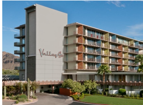
Hotel Valley Ho on Main Street in Old Town Scottsdale
