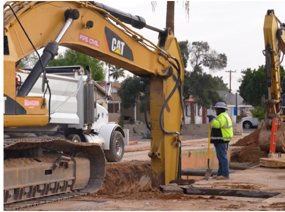
Construction is underway on the Roosevelt Street Storm Drain Project.
