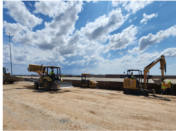
Loop 101 project under construction
