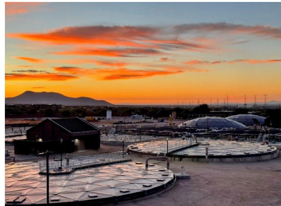
The sun sets over Scottsdale's Advanced Water Treatment Facility.
