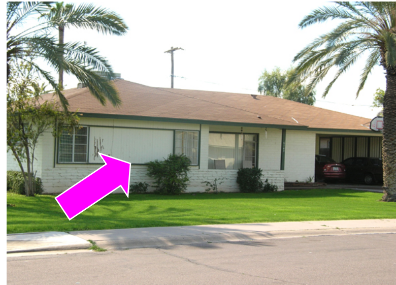
Horizontal wood panels were used between the two windows on the L-end to vary the appearance.
