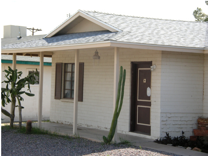
Entry doors were located under small porch roofs. This model has the door facing the street and is located on the L-end of the home, under a porch roof that is supported by four wooden posts.
