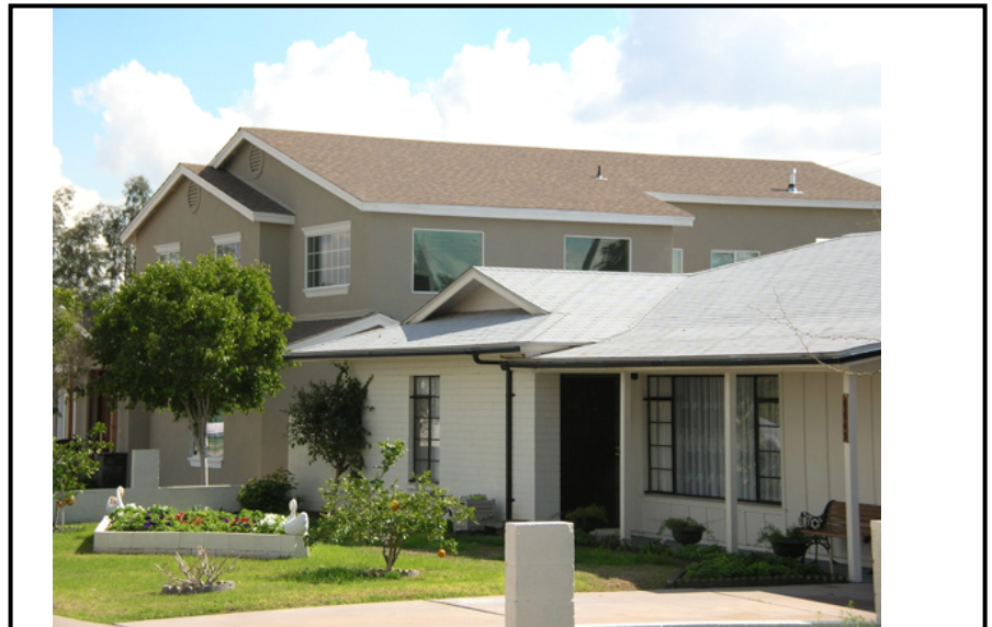
A new taller two-story home, set back the same distance from the street as adjacent homes, looks out of scale relative to the surrounding one-story homes that have a more horizontal emphasis.
