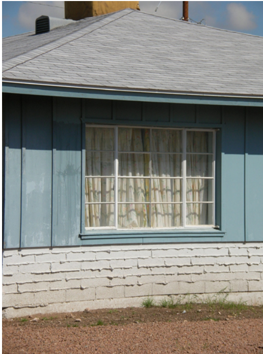
The original steel casement windows used in Ranch style homes have a variety of types and pattern. The above windows has sixteen rectangular shaped panes and the side windows can be cranked open.
