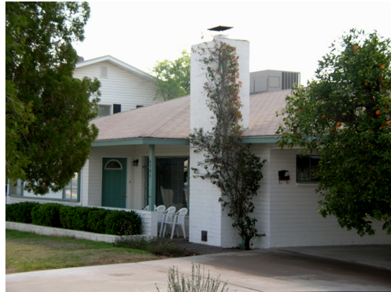
Chimneys should be placed on the side of the house or they could protrude through the roof at the ridgeline or behind the ridgeline. Avoid chimneys on the front façade.
