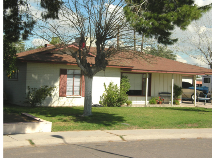
Allied used L-shaped floor plans and varied the appearance of the L-end of the front façade. The above Simple Ranch style home has the L-end projecting out in front of the rest of the façade and a modified hip roof.
