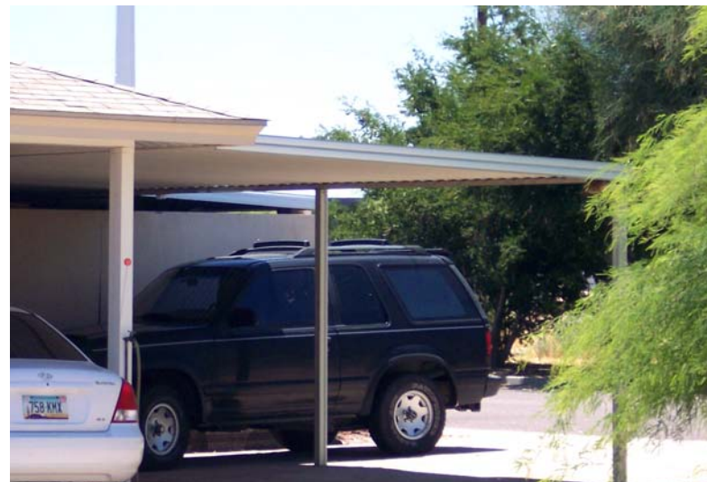
A metal carport addition with a flat roof and metal posts is not appropriate for the area.
