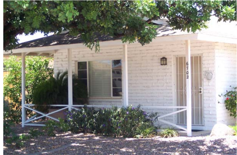
All of the original features of this porch on the L-end of a Village Grove home appear to have been maintained – the modified hip roof, the square wooden posts, and the western style railings.
