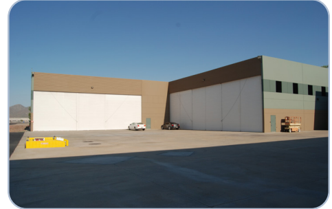
Hangars generally require larger building mass, fewer parking spaces, and less open space than other land uses.
