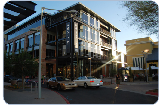
Locate offices within walking distance of restaurants and shopping to promote a convenient working environment.
