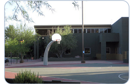
Facilities, such as Horizon Community Center, can provide meeting space in addition to recreational activities.
