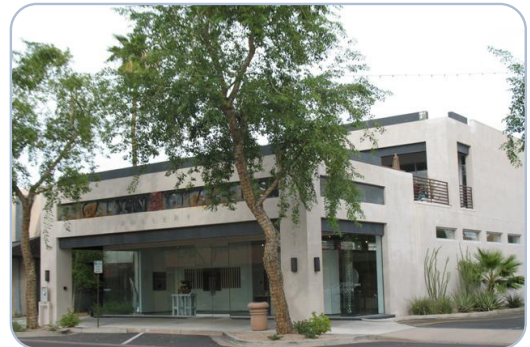
Building stepback is another possible solution to sensitive edge buffering.
