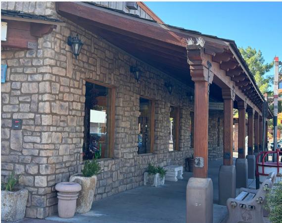
The clear glass windows of this retailer are deeply recessed into the stone wall, providing a sense of the wall massing.
