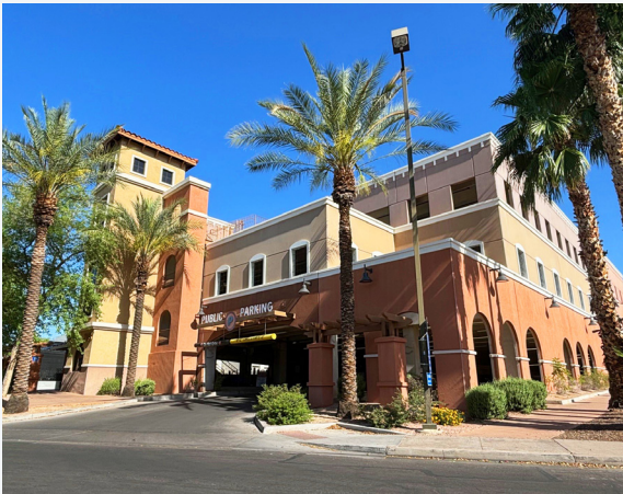
Minimize the apparent mass of a parking structure through building design and architectural features, setbacks, and building articulation.
