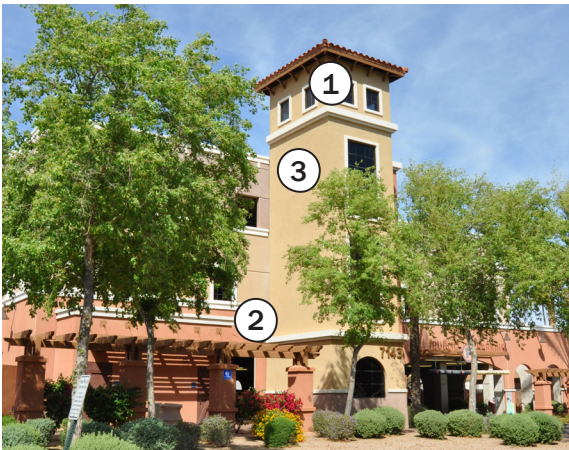
5th Avenue public parking garage.
