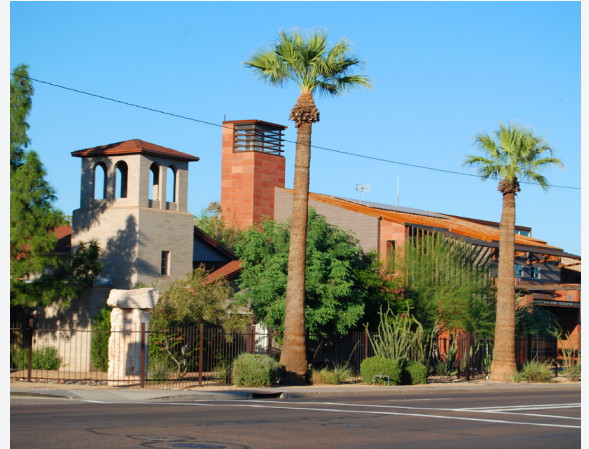
The balance between the new building design of the fire station with the existing church design (foreground) is strengthened by shared features such as concrete block as a key material, tower and roof features with similar geometry, similar roof pitch, street continuity, and metal picket fencing.
