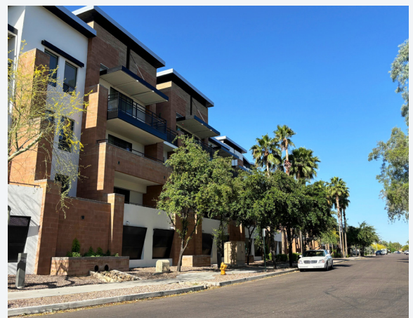
DISCOURAGED - Podium parking with no active uses at the street level.
