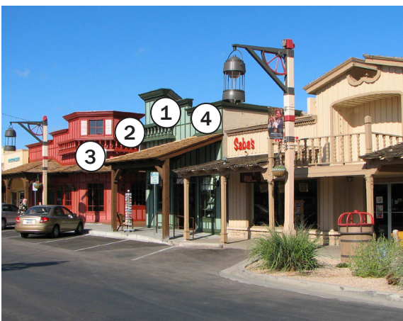
Old Town street frontage.
