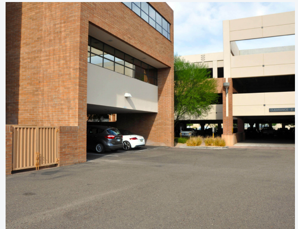
A single parking bay incorporated into the building design, and internal to the site, beneath the second floor.
