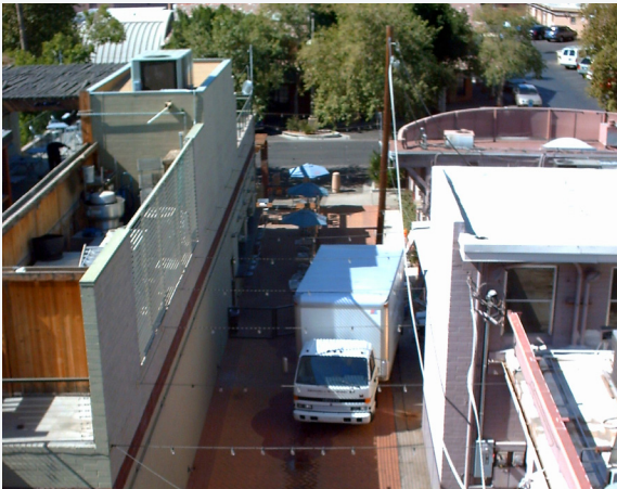
ENCOURAGED - Alley service/deliveries and screened building equipment.
