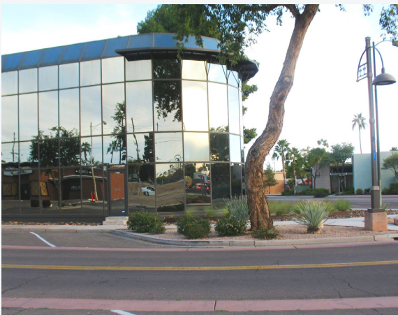
DISCOURAGED - The mirrored glass clad building lacks transparency, causes glare, and does not project a desert southwest character or sense of place.
