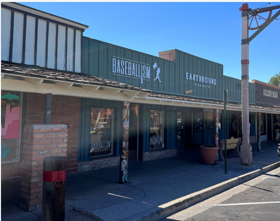
This storefront incorporates a traditional style covered walkway, wood-frame windows, and a brick wainscot below board and batten siding. The storefront has multiple entrances and doorways that are recessed as well as decorative, Western details.
