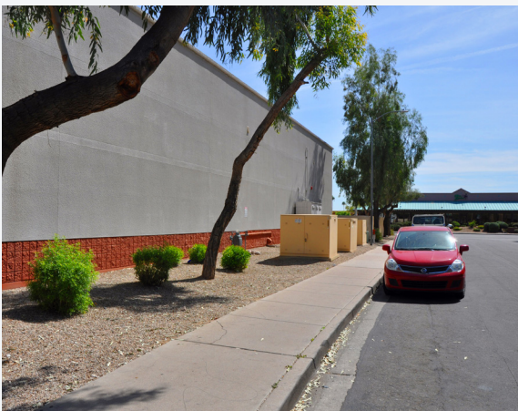
DISCOURAGED - Unscreened electrical equipment and blank building wall facing a public street.
