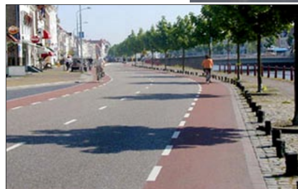
Color treated asphalt (“Asphacolor”) - example from the Netherlands
