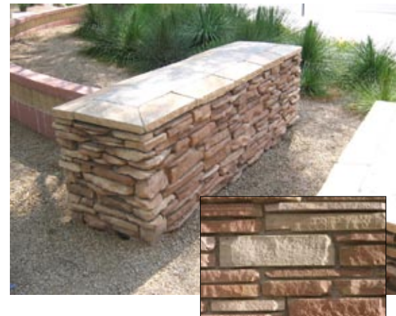
Dry Laid Sandstone
