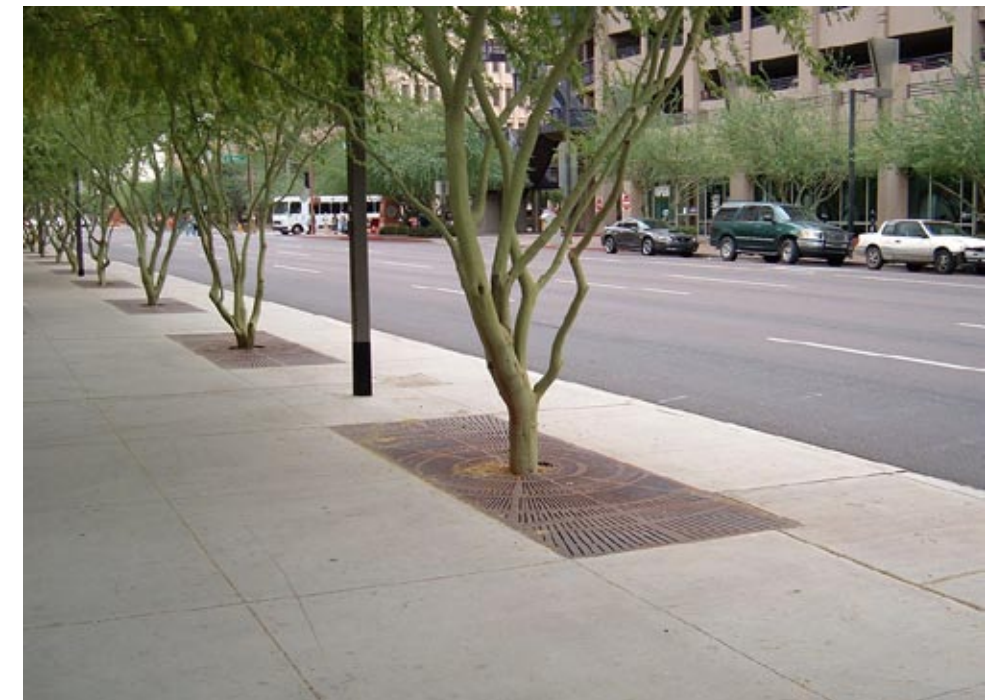
Tree grates will be used near bus stop areas and at intersection corners to maximize sidewalk capacity and accessibility. The tree grate design will be consistent with the steel cut-out pattern selected for each segment
