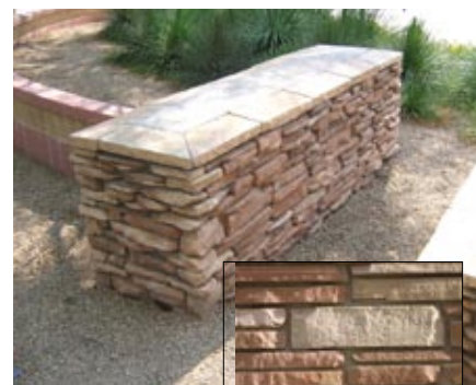
Dry Laid Sandstone
