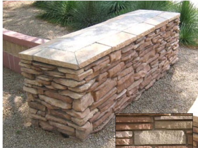
Dry Laid Sandstone
