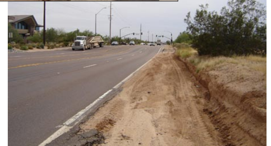
Examples of graded shoulder and utility cabinets in Segment 5 and 6
