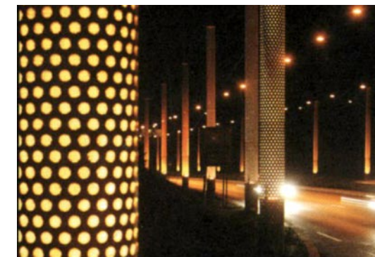
Light pole wraps to match decorative metal panels for the Segment 2 (Homestead)
