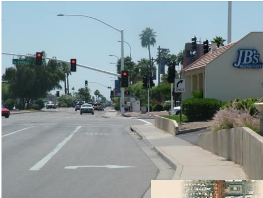
Additional right turn lanes in Segment 1 reduce the amount of space in the right-of-way at McDowell Road for pedestrian and bicycle facilities
