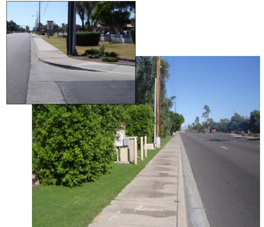
Sidewalks are present in Segment 3, but are often narrow with utilities located directly adjacent to them
