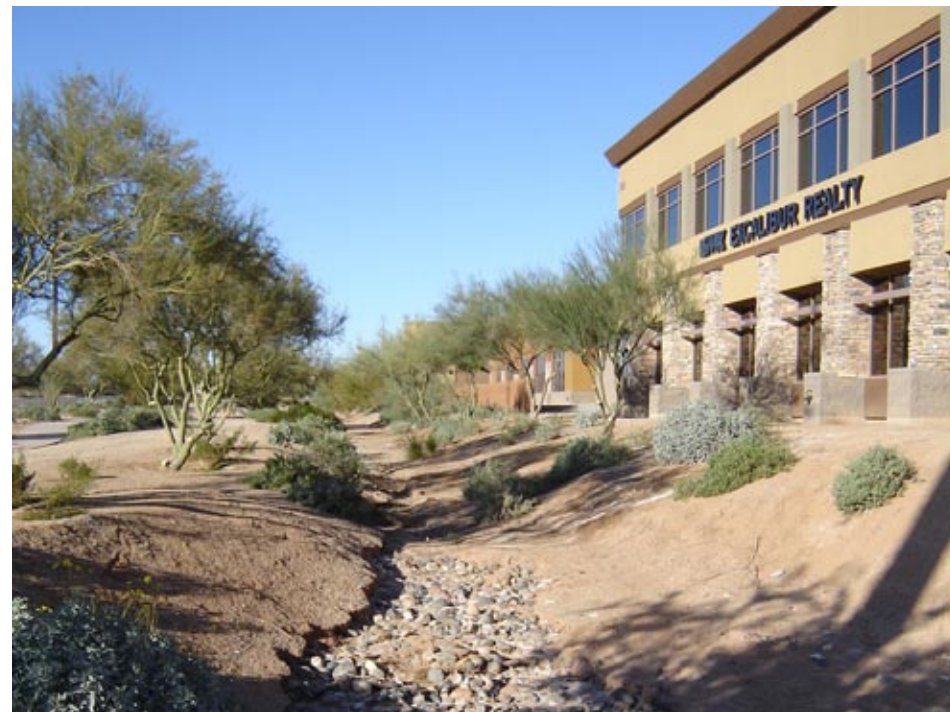
Washes run throughout the area sometimes crossing paths and the roadway
