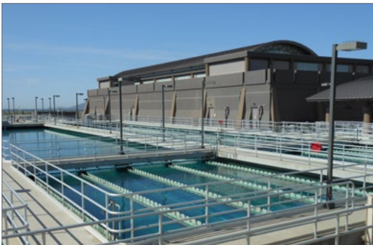
Scottsdale's CAP Water Treatment Plant
